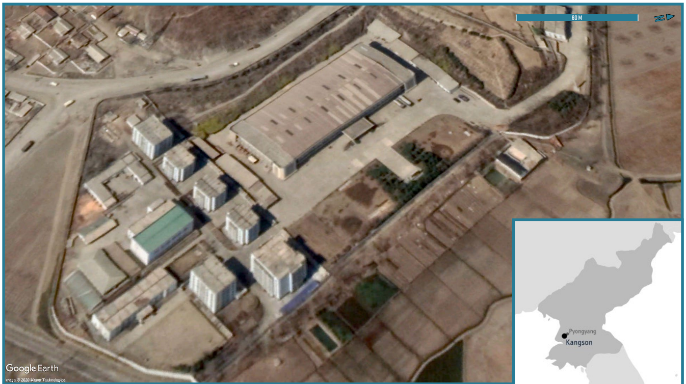
▲ FIGURE 3 The facility known as Kangson has been identified as a possible location of a uranium enrichment plant. (Google Earth)
