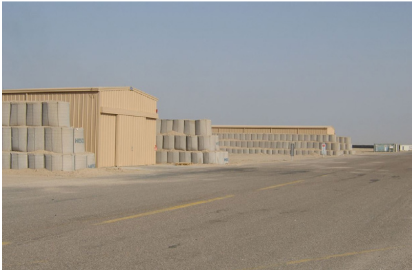
Figure 22 – Barricaded Light Walled Frangible Ammunition Storage Solution. 102)
