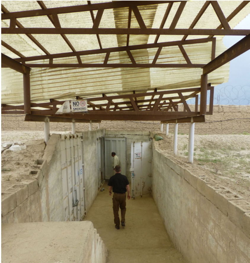
Figure 7 – Environmental Protection on Shipping Container Based Ammunition Storage. 50)
