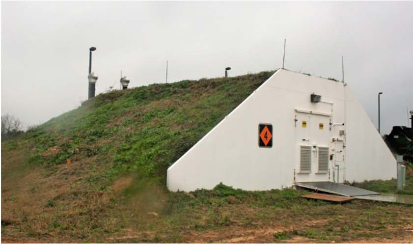
Figure 25 – Pre-Fabricated Metal Earth Covered Magazine - As Built. 105)
