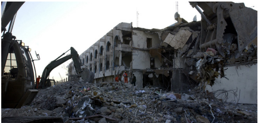
Figure 3 – Aftermath of the Bombing of the UN Headquarters in Baghdad, Iraq. 7)
