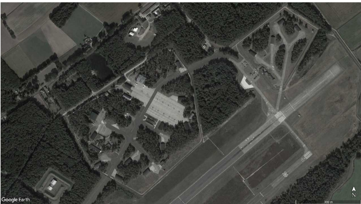
Figure B4. Former Quick Reaction Alert site (upper right) and igloo-type storage area (left side) at Kleine Brogel
