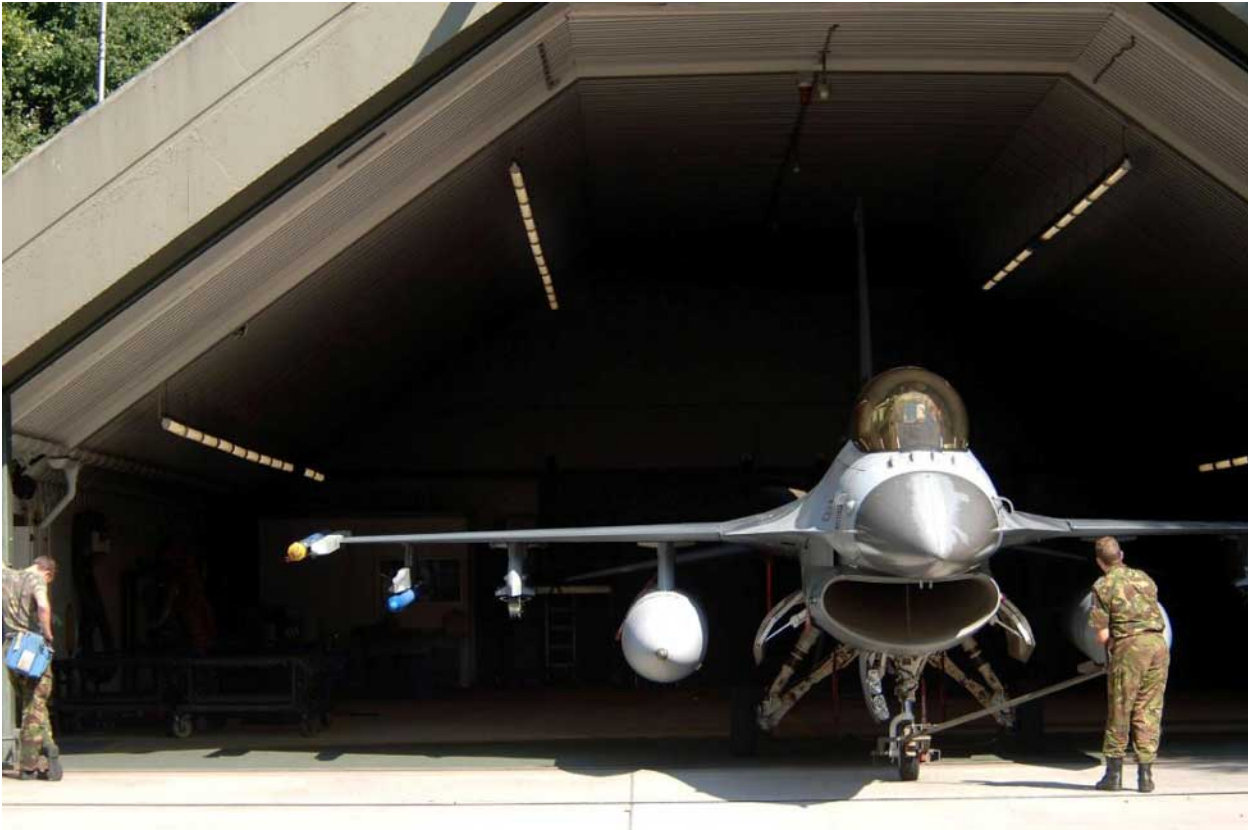
Figure B1. Protective Aircraft Shelter at Volkel Air Base in the Netherlands. (Source: US Air Force)
