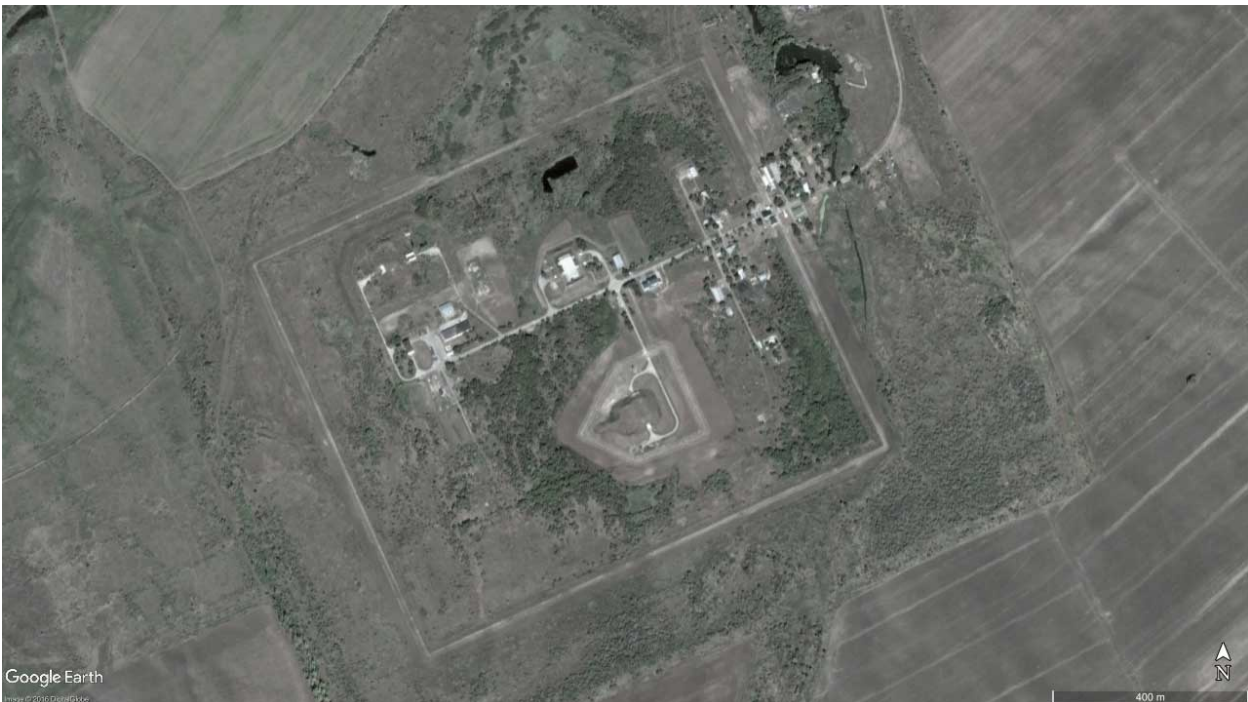
Figure A4. Base-level storage facility at Engels air base
